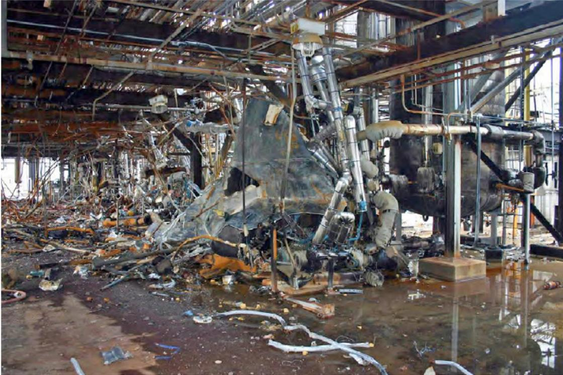
Figure 3. Path of destruction caused by careening residual treater vessel, which came to rest as shown in the center of the picture (from CSB 21 April 2009 report). The residual treater is designed to decompose waste methomyl in a solvent carrier before final incineration.
