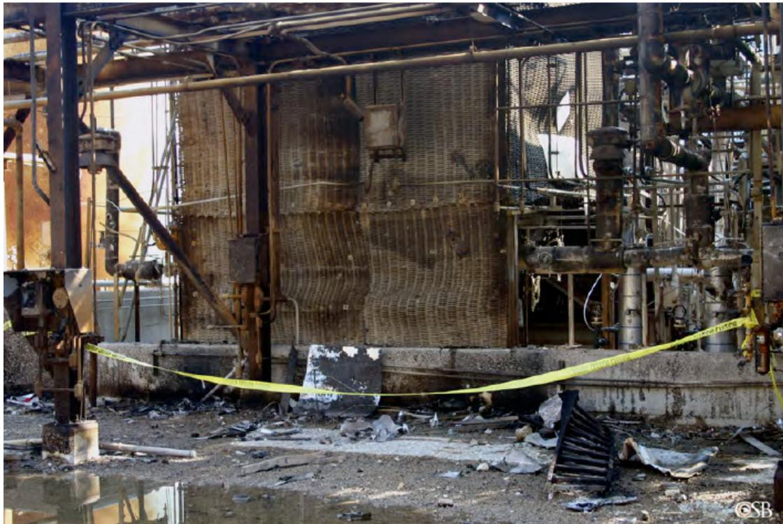
Figure 2: The blast blanket protecting the MIC tank. Note explosion debris in the foreground. Both illustrations from the CSB report on 21 April 2009 to the House Committee cited earlier.
